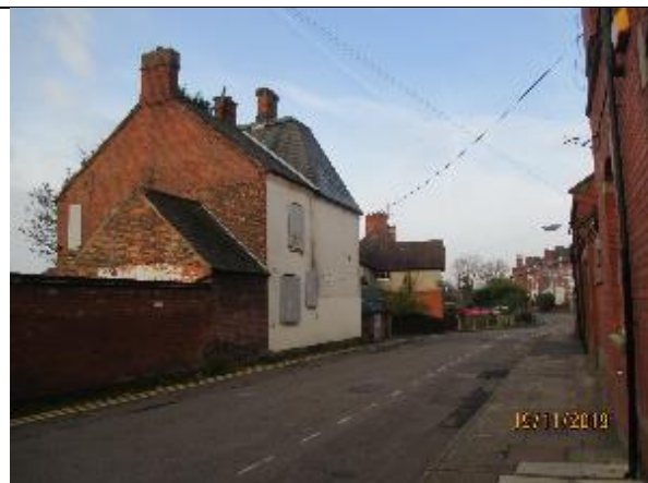
North west elevation of the Gatehouse
