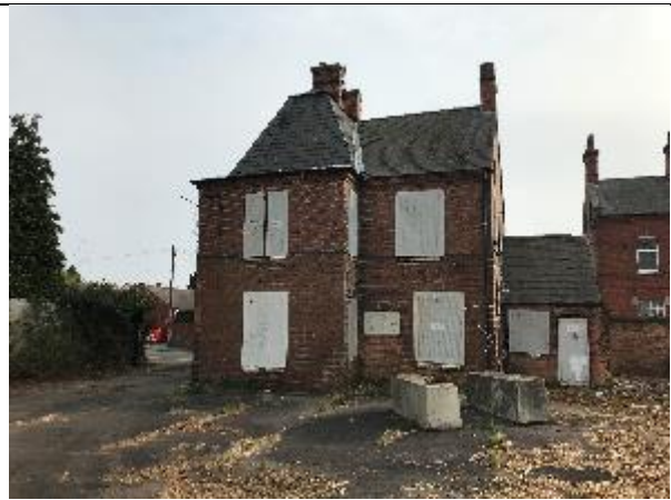
Rear (north east) elevation of the Gatehouse
