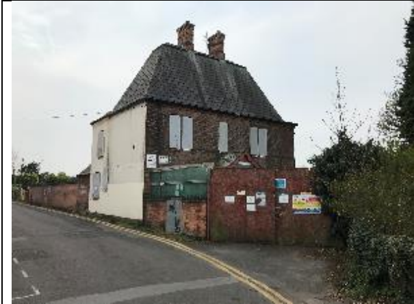
South east elevation of the Gatehouse
