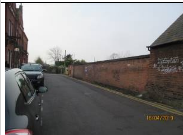
Existing boundary wall to the site
