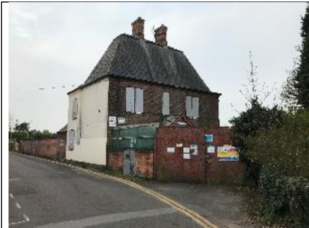
South east elevation of the Gatehouse
