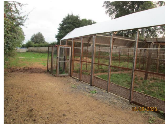
Exist' Existing enclosure
