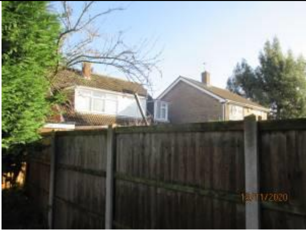
Rear elevation of 2 Rookwood Close
