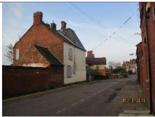
North west elevation of the Gatehouse
