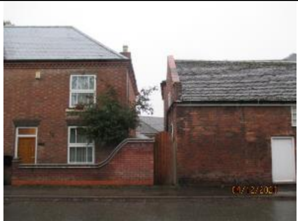
Gap between 259 and the adjacent home, site of the proposed link building
