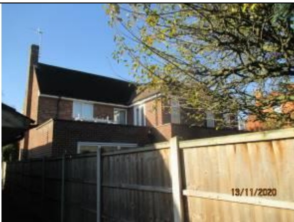
Rear elevation of 34 Park Road
