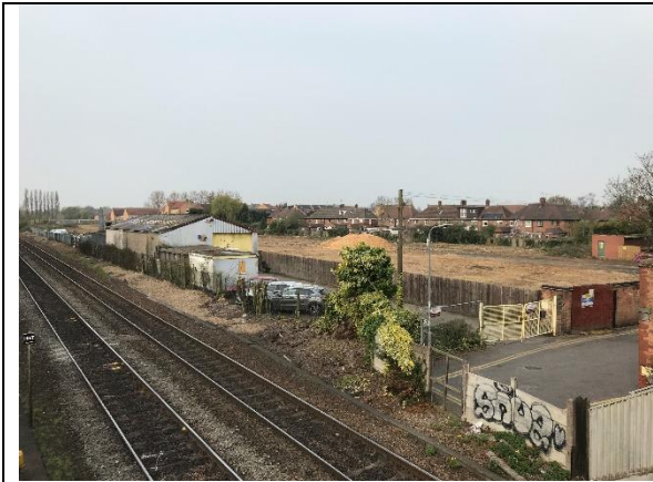
View from railway bridge, looking south west
