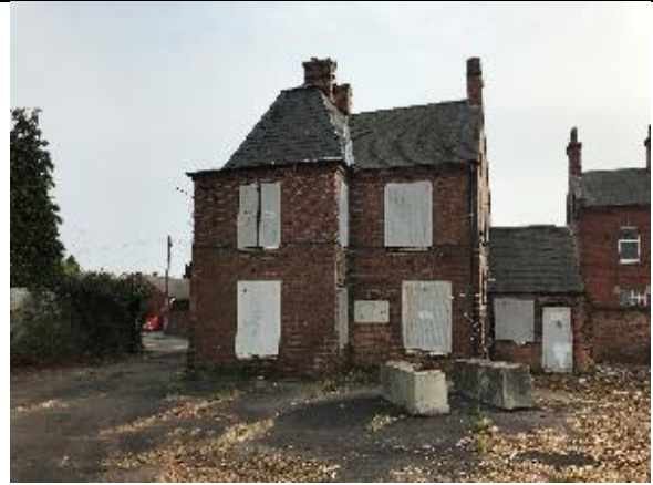
Rear (north east) elevation of the Gatehouse
