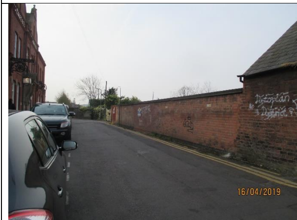
Existing boundary wall to the site
