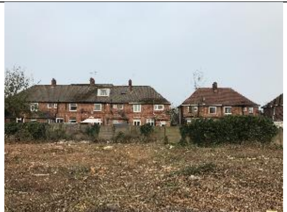
Rear of properties on Redwood Crescent, which are to the north west of the site
