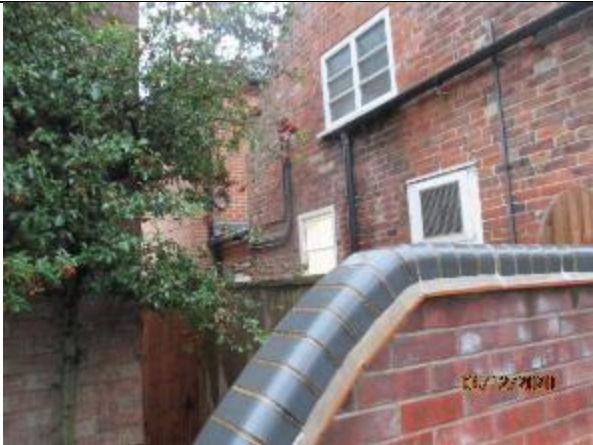
North east elevation of the adjacent building. The link would be to the flat roof element that can be seen to the rear of the adjacent building
