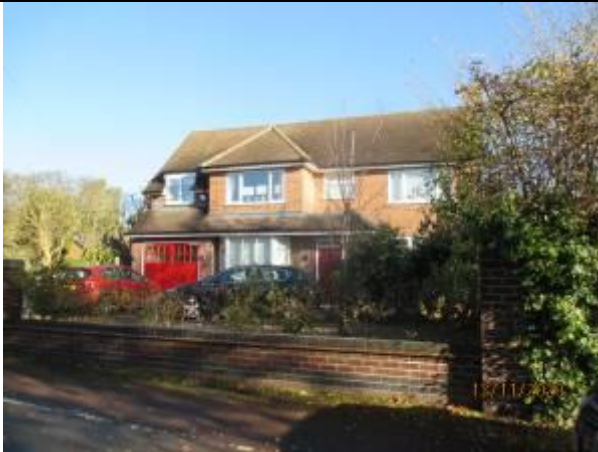
Front elevation of 34 Park Road
